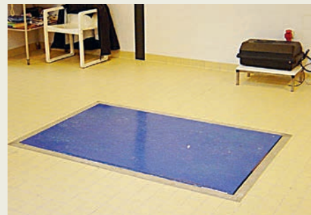
Lift table installed in a pit.
