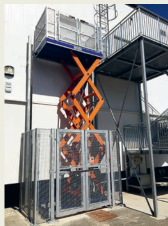
Goods and freight lift
